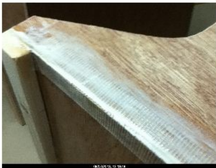
Finished taped edge
