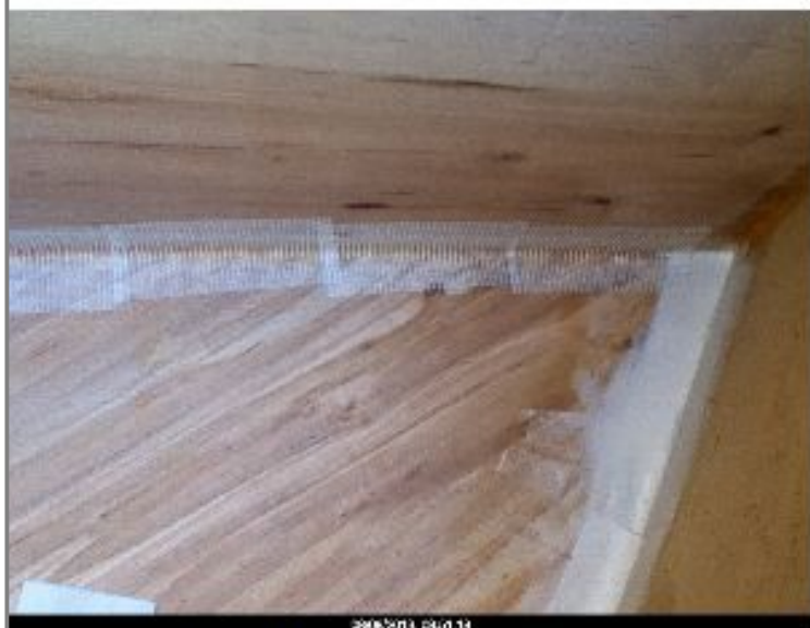
Overlapping Taped Sections
