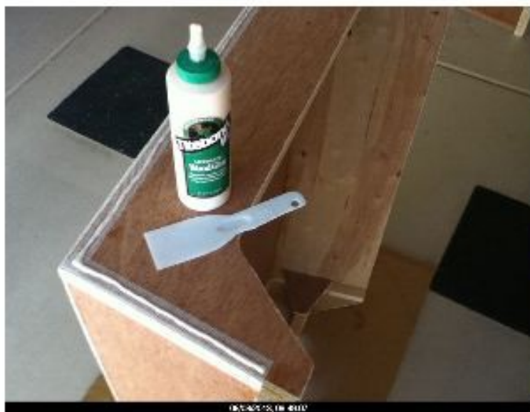
Typical glue bead size
